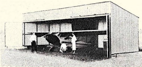
Easily transported and capable of being assembled by two men in a few hours time, this low cost metal hangar will provide ample storage space for the average small airplane.
