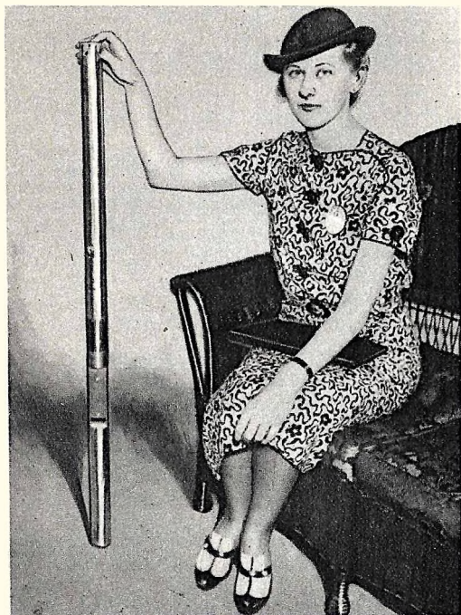
The stake-like affair held by Miss Ann Hollenburg, and demonstrated at the recent Tulsa, Oklahoma, Oil Exposition is the new power-driven, electric-lighted oil well camera.
