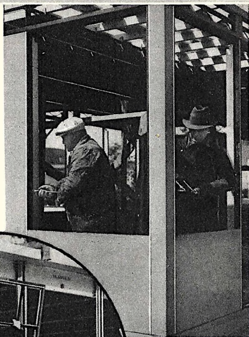
General Houses, Inc., are pioneers in the development of the pre-fabricated steel panel and steel frame house, which are put together with a socket wrench. They have just introduced new model homes to sell from $2,500 to $5,500. These houses are built in 2-foot sections.
