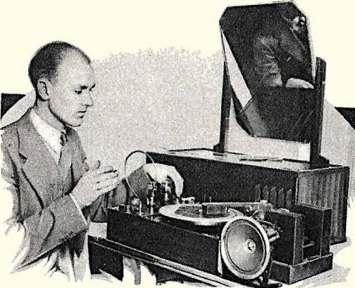
Anyone pausing to inspect himself before this mirror is rewarded with a sales talk delivered by automatic phonograph shown in the foreground. An electric eye starts the machine.
