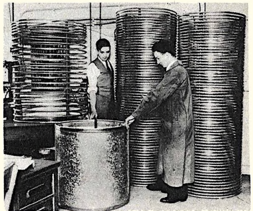
Dr. D. B. Paarkinson, left, and Dr. R. G. Herb of the University of Wisconsin, shown inspecting power plant of a new atom gun expected to develop a potential of 2,500,000 volts.
